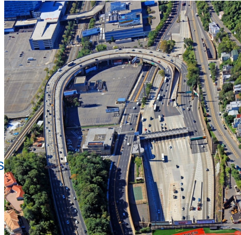
View of Existing Helix Planned Construction 2020-2025
