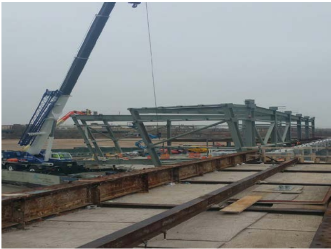
Existing Westbound platform, construction new Northeast Head House
