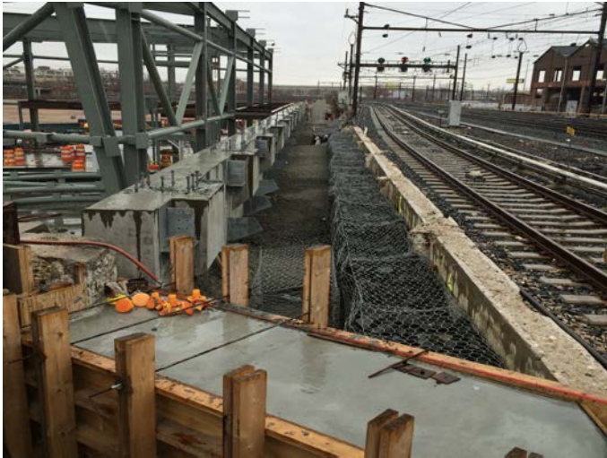
Westbound platform, installation gabion baskets, extension to east abutment wall
