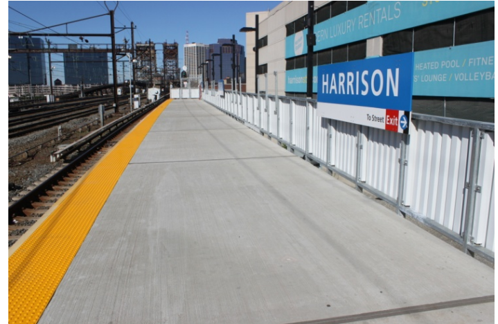
Temporary Platforms Installed
