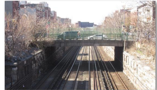
East 188 th Street Bridge
