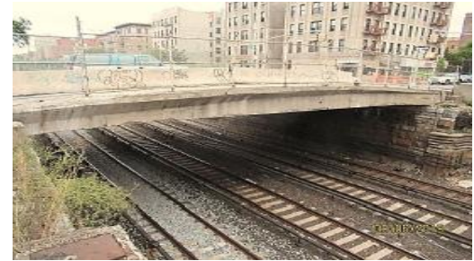
East 183 rd Street Bridge
