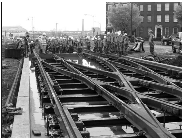
Cadets inspecting NERL special trackwork.
