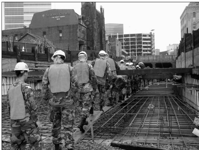
Cadets enter the new NERL tunnel.
